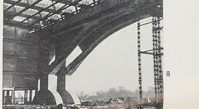
7. 8. United Airlines hangar at San Francisco International, by Skidmore, Owings and Merrill; interior of BOAC hangar at London Heathrow. Major monuments of the structural engineer's art—Sir Owen Williams at San Francisco, Sir Owen Williams at Heathrow—but all too often buried in marginal suboptimal
